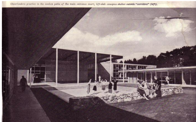
Cheerleaders practice in the sunken patio of the main entrance court; lift-slab canopy shelter outside "corridors" (left).
